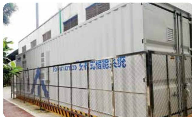
Location: Dongguan,China Capacity: 500kW/1.5MWh Model: BD500KTR-T
