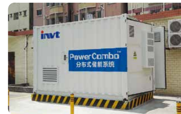
Location: Dongguan,China Capacity: 500kW/300kWh Model: BD500KTR
